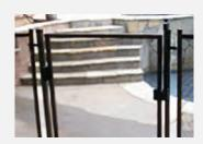
**Single Pole Truss with Reinforcement Bar:** The same as above, however they add a bar across the 1st two fence sections to make up for the weakness of the gate. This also adds a staging platform for a child to get a foothold. The latch is within a child's reach.
