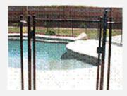
**Single Square Stock:** Still a single truss attaching to the fence. The advantage is the latch and hinges sit on a flat surface only on one side. The disadvantage is the gate is made of fence poles and has no top support on the gate other than the fabric. It also has a bar across the bottom, creating a trip hazard going into the pool area. This type of gate is put together by the installer, not the manufacturer, and the mesh is only bordered at the top.
